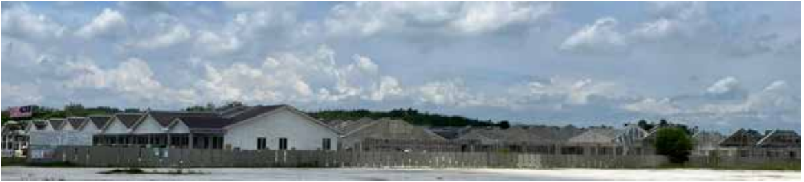
Sri Iskandar's terrace houses in progress
